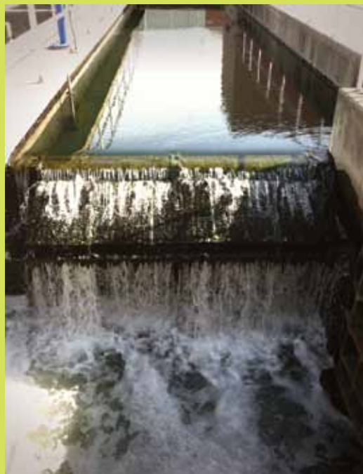
The plant's cascade structure, which allowed it to meet the minimum NPDES DO requirement.
