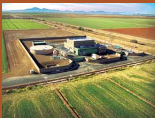
An aerial view of the Ak-Chin Indian Community surface water treatment plant, taken from an ultra-light aircraft by Dave Weesner, superintendent for PCL Constructors
